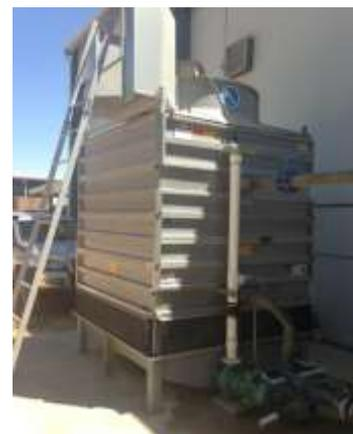
In order to keep the ammonia charge of the package to a minimum Alfa Laval PHE are used for condensers and oil cooling (Figure 7), water is circulated through a close loop through a BAC fluid cooler (Figure 10) and pumped through both PHE's.
