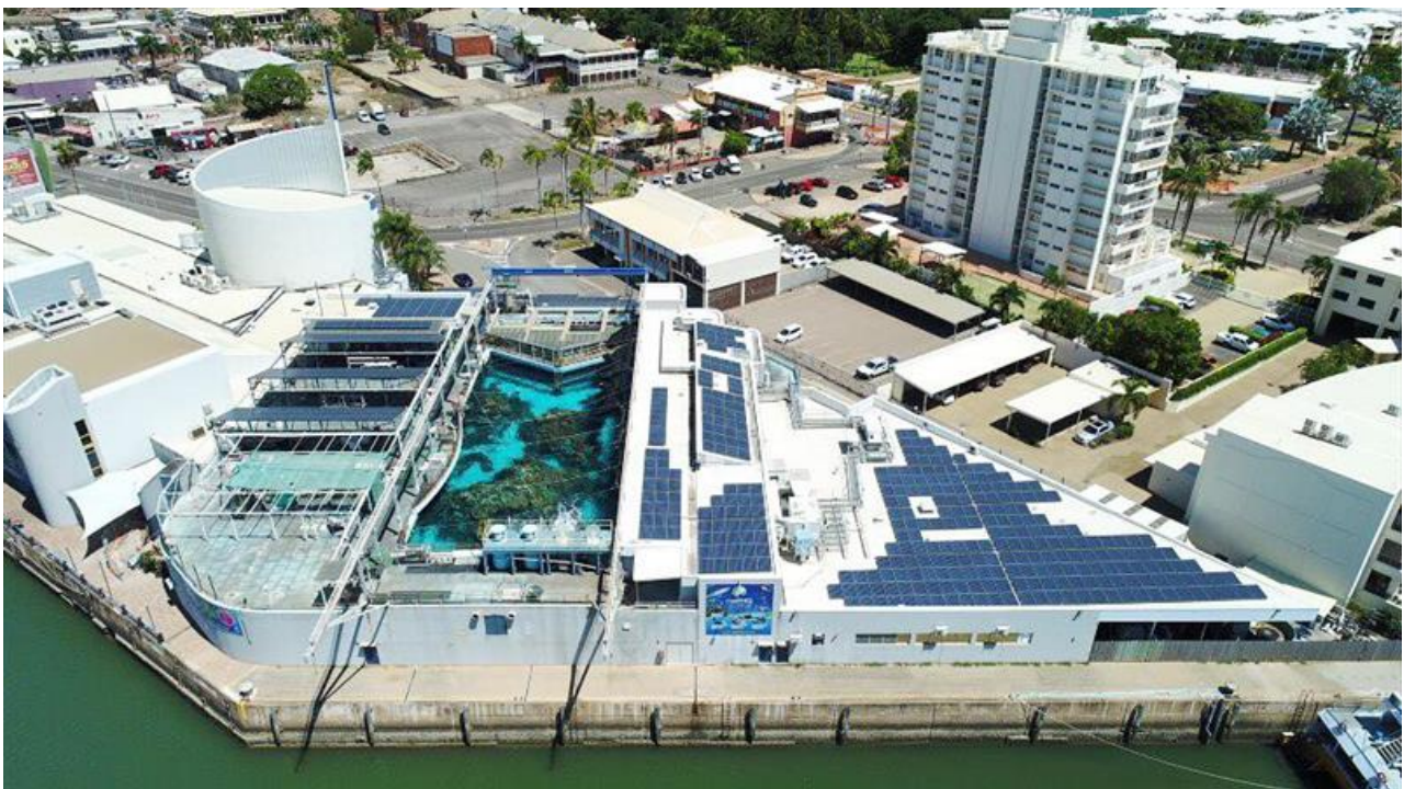
The existing solar system at the Reef HQ Great Barrier Reef Aquarium in Townsville. Image: Commercial Drone Photography
